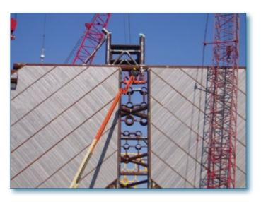
FRP structural shapes, including FRP Mud Mats, have 2 components of deflection. A flexural component and a shear component due to the fact that FRP structural shapes possess a low Shear Modulus, G, of only 500,000 psi.
